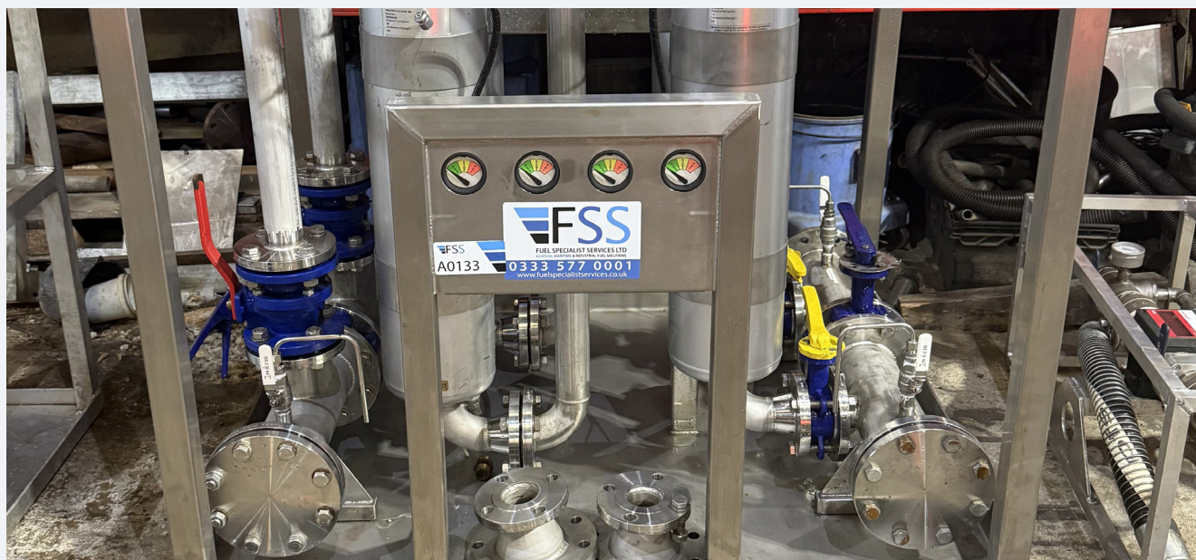
Stand-alone automated duplex fuel polisher for install on existing fuel tank
